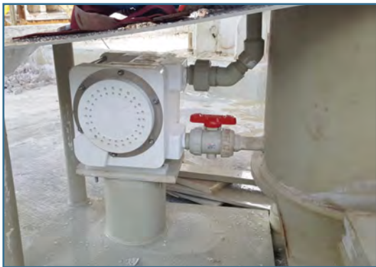
QUANTUM pump installed for HF transfer to reactors (Italy)
