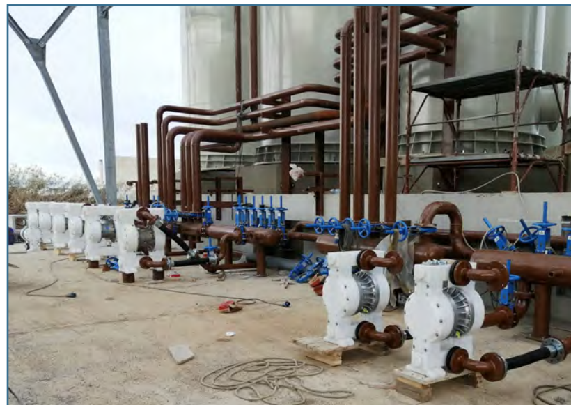
ASTRAsolid pumps (2") installed outside the plant, nearby the coastline for polluted and waste treatments (Italy)
